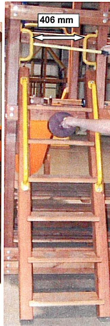
Conclusion: The exit entrances on both opening must be more than 500-mm width of entrance and exit openings in barriers shall have a clear opening of 500-mm maximum unless a guardrail is provided across the opening. The rockwall entrance and exit openings measure 457-mm (18") and the step ladder opening measures 406-mm (16").
